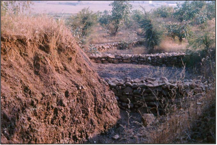
Above: Loose boulder check dams on the nala on the west side of Patni village; and below: A tank built on the south side of the village.
