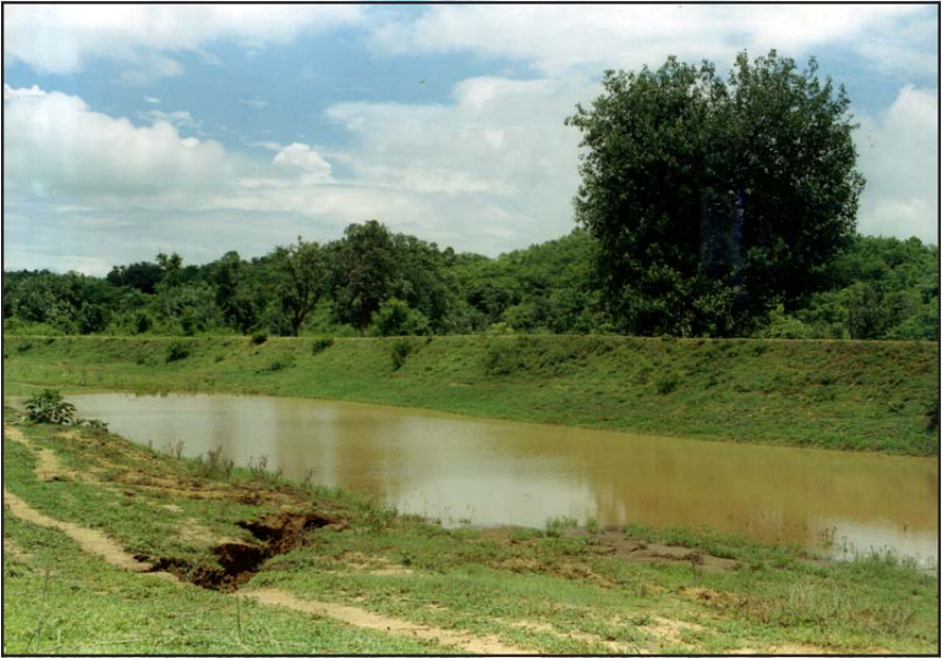
Above: The bund of a percolation tank with ground water seepage at Tagi; and below: in-situ field bunding for moisture conservation in Majhgawan.
