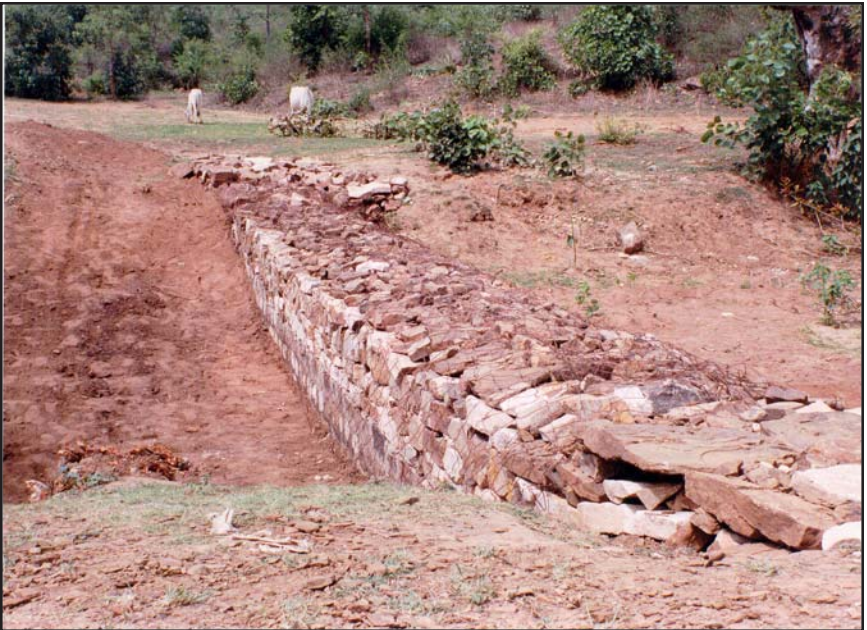
Above: A loose boulder check dam at Chitauriha; and below: A Gabion structure at Majhgawan.
