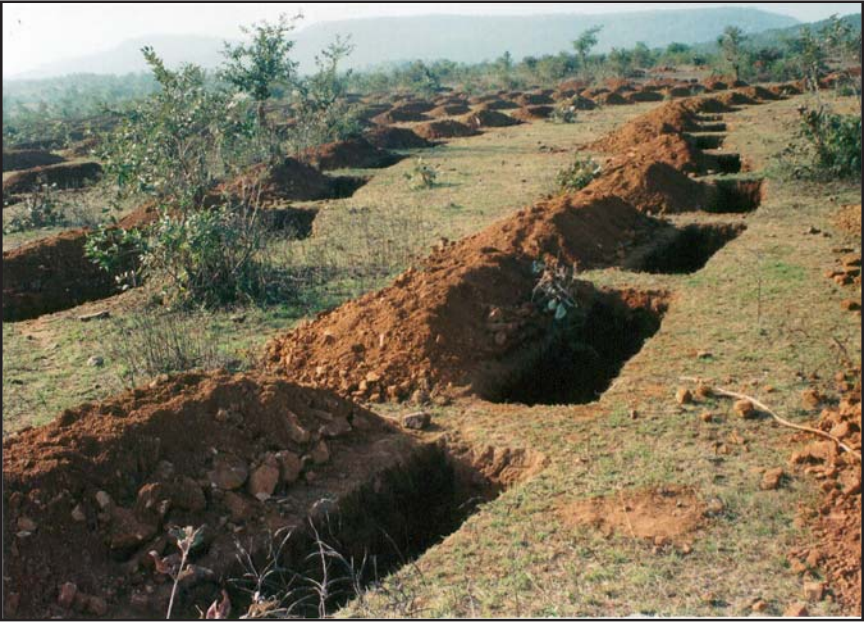
Above: Contour trenches at Patni; and below: Stone pitching on earthen bunds at Khodari.
