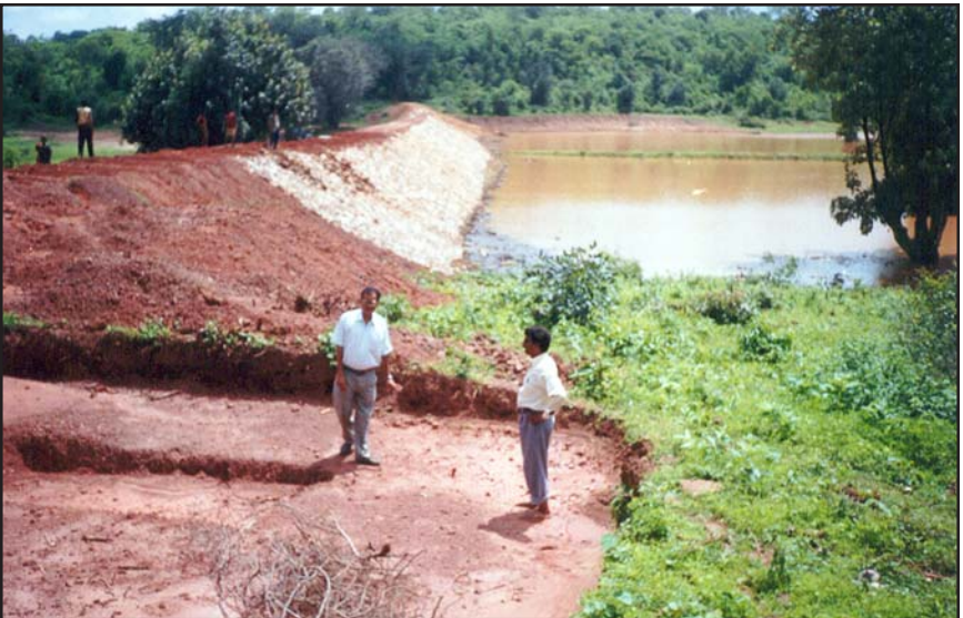
Above: A cattle-proof trench at Kavar; and below: A side spillway at zero level, Khodari.
