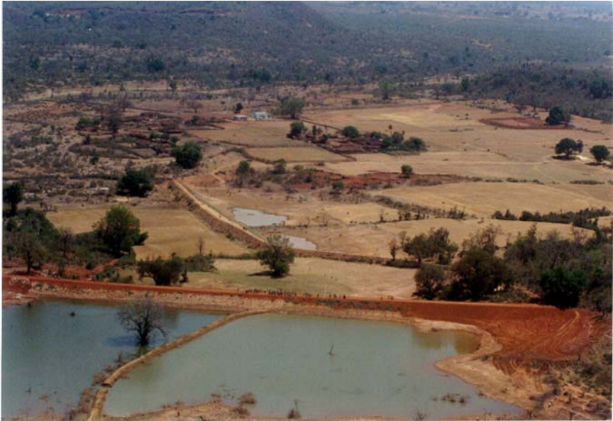
Earthen nala dam with side spillway, Khodari.
