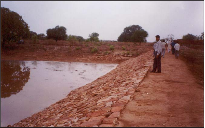
Above: Contour trenches at Patni; and below: Stone pitching on earthen bunds at Khodari.
