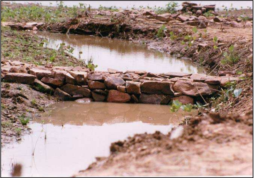
Above: A loose boulder check dam at Chitauriha; and below: A Gabion structure at Majhgawan.
