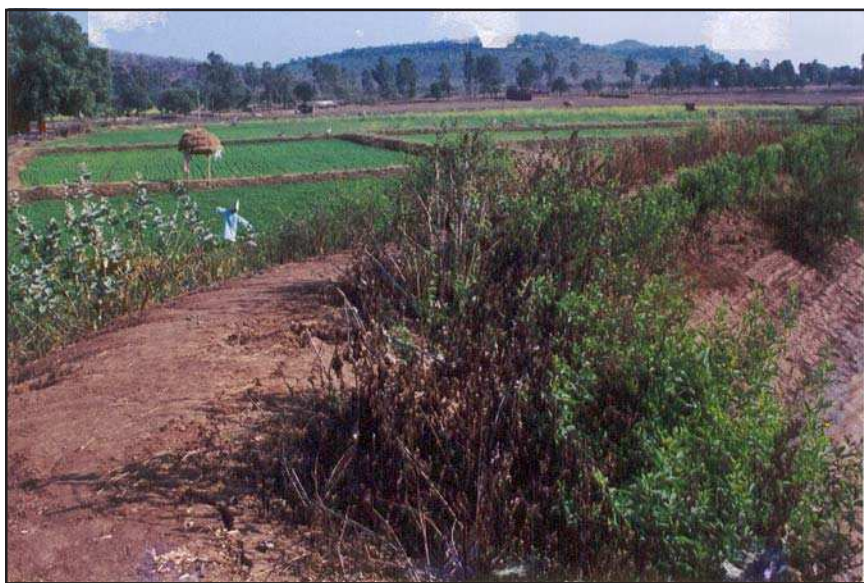
Above: The bund of a percolation tank with ground water seepage at Tagi; and below: in-situ field bunding for moisture conservation in Majhgawan.
